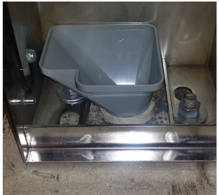
Coin chute installed in a poured pedestal.
