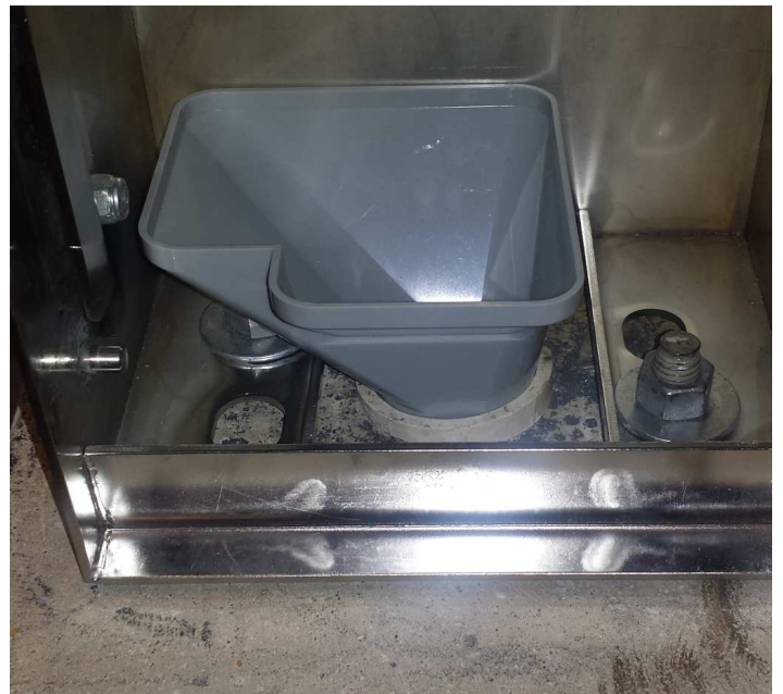
Coin chute installed in a poured pedestal.
