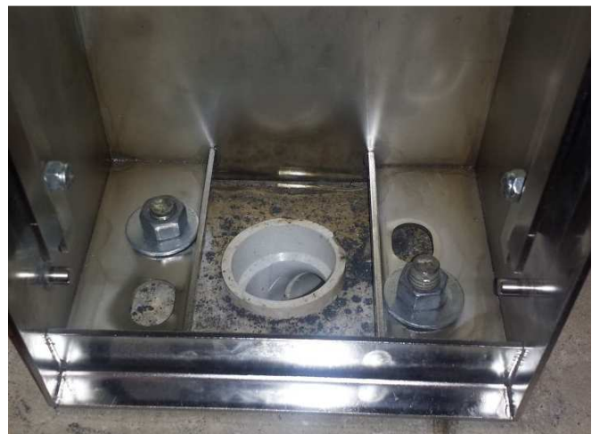
Complete the tower installation using two washers and nuts as shown.
